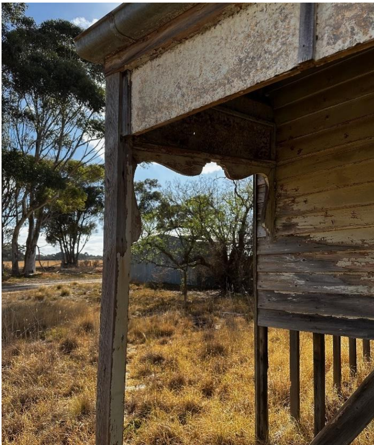
Photo 12: Verandah at the front of Closer Settlement Homestead 1
