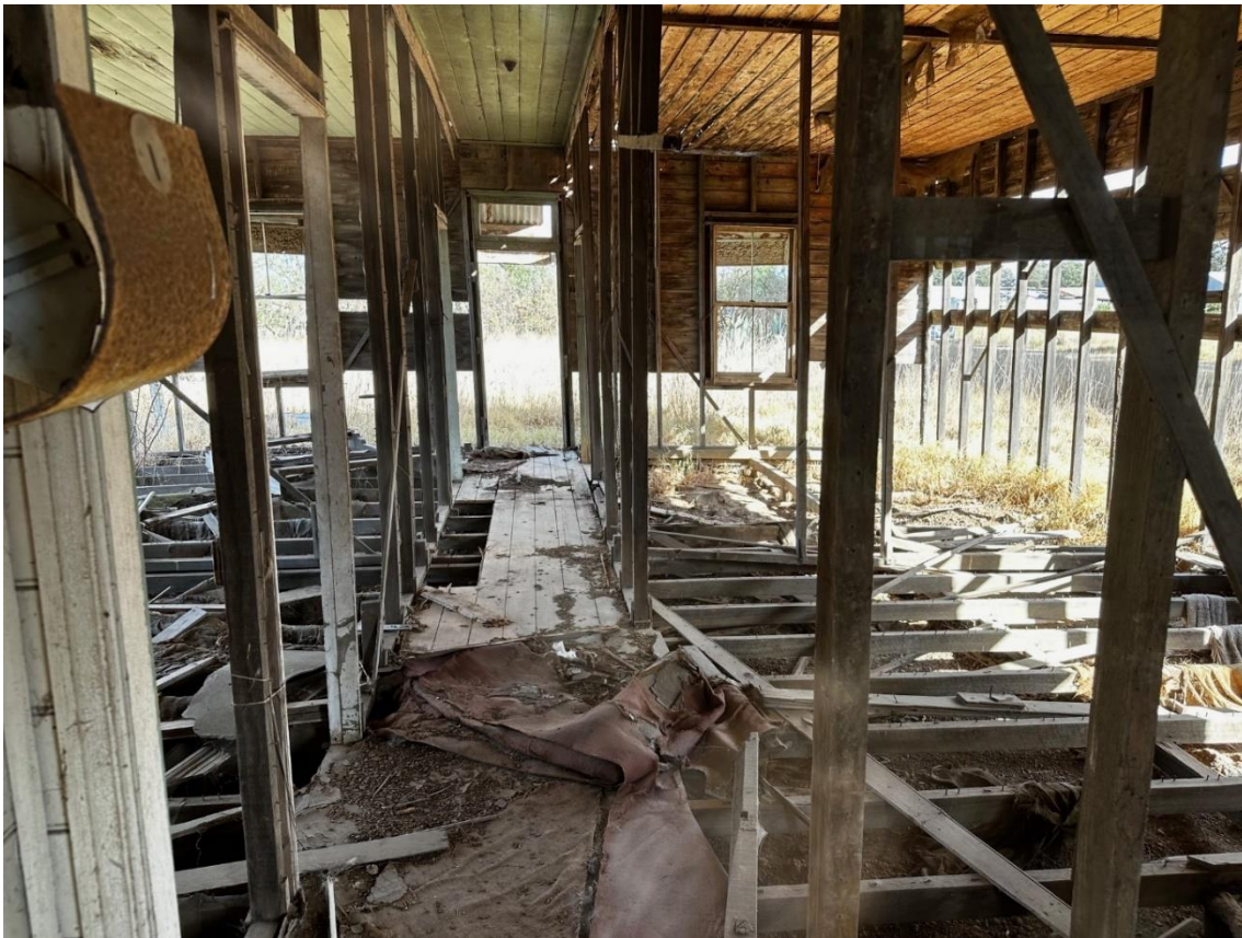
Photo 13: Hallway and rooms inside Closer Settlement Homestead 1
