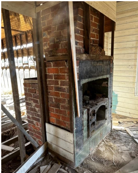
Photo 14: Kitchen stove and chimney at Closer Settlement Homestead 1
