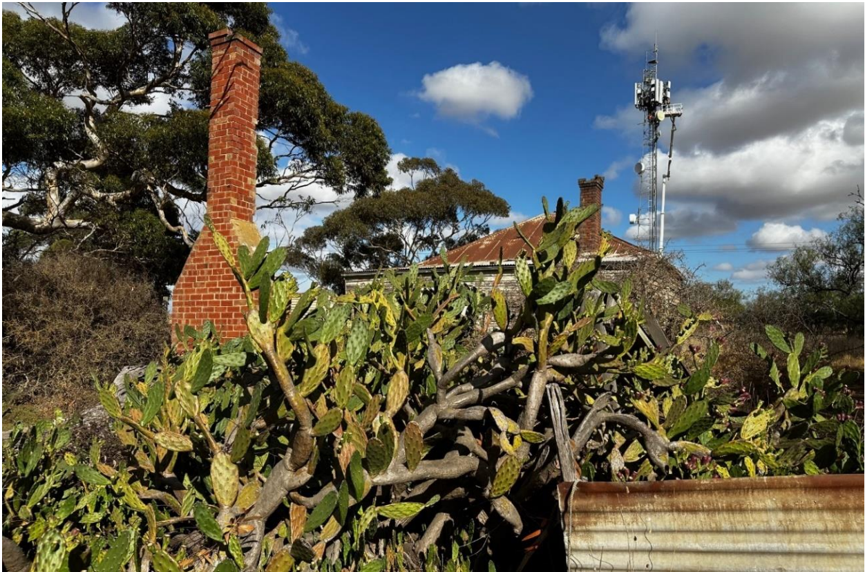
Photo 9: Rear view of Closer Settlement House 1 showing extant shed chimney
