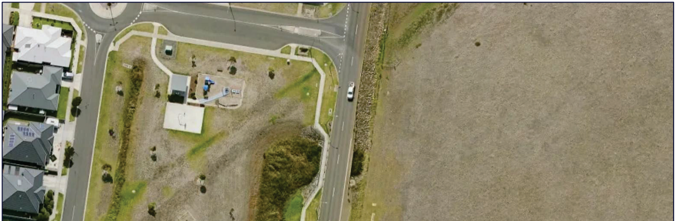
Existing Aberline Road Culvert Crossing
