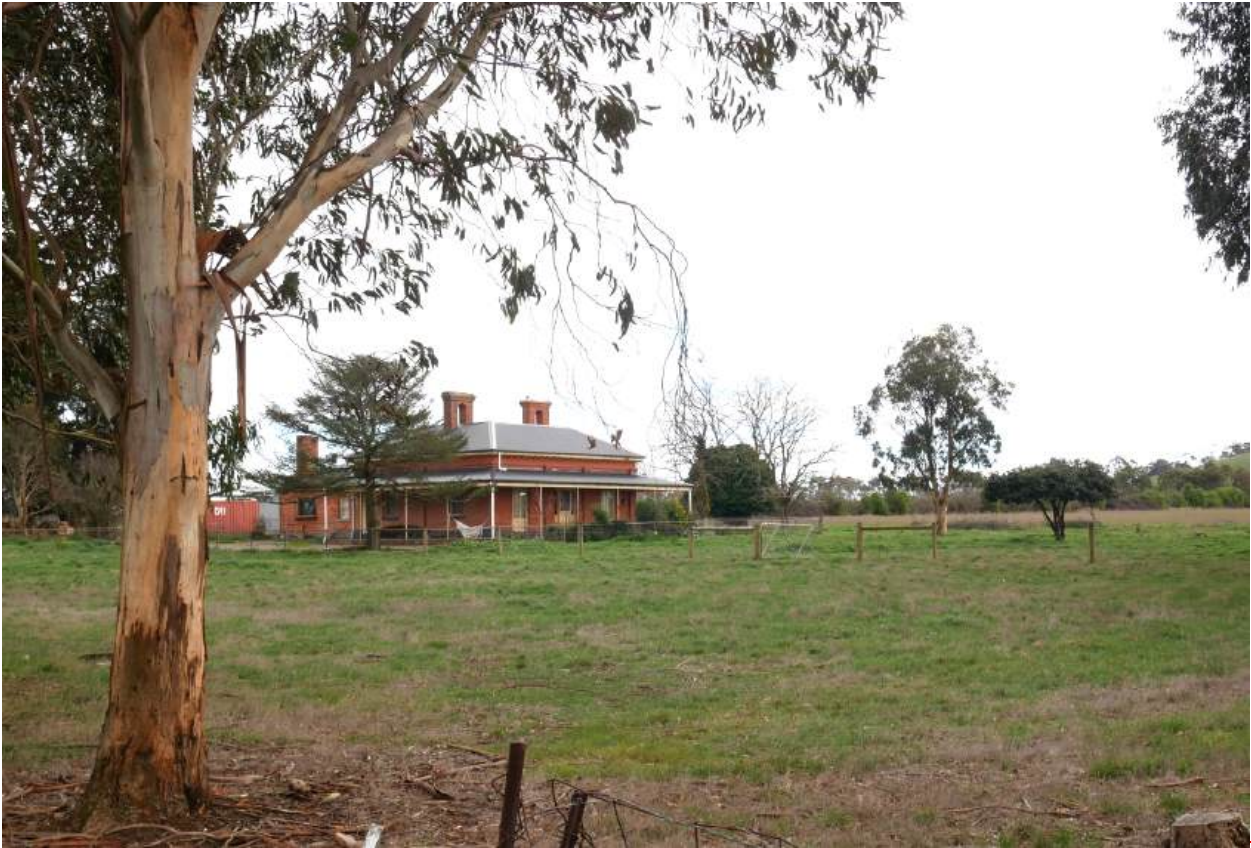
Figure 1. Bernera Homestead from Olliers Road. (Source: GJM Heritage, August 2025)
