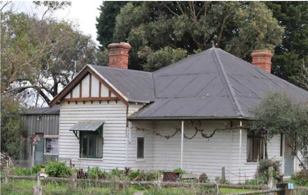
Figures 1 and 2. Homestead at 103 Olliers Road – front (north) elevation and east (side) elevation. (Source: GJM Heritage, August 2025; RBA, August 2024)
