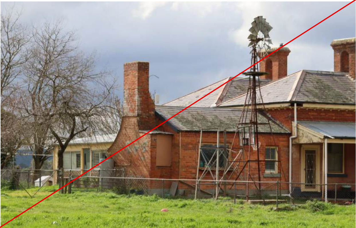
Close-up of the original secondary rear wing with the skillion-roofed addition in the background.— (Source: RBA, August 2024)
