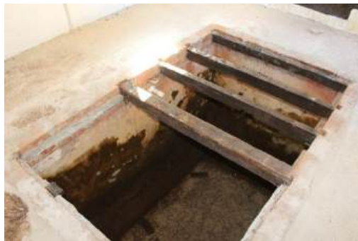
Figure 12. (Above) 'Pit', floor of the creamery outbuilding (Source: RBA, September 2023)
