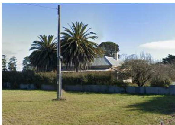
Figure 11. 624 Glenelg Highway, Smythes Creek (Source: Google Street View)
