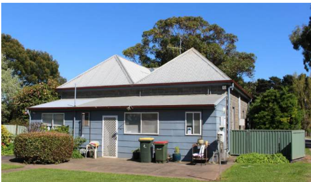
Figure 10. Rear (west) elevation (Source: RBA, September 2023)
