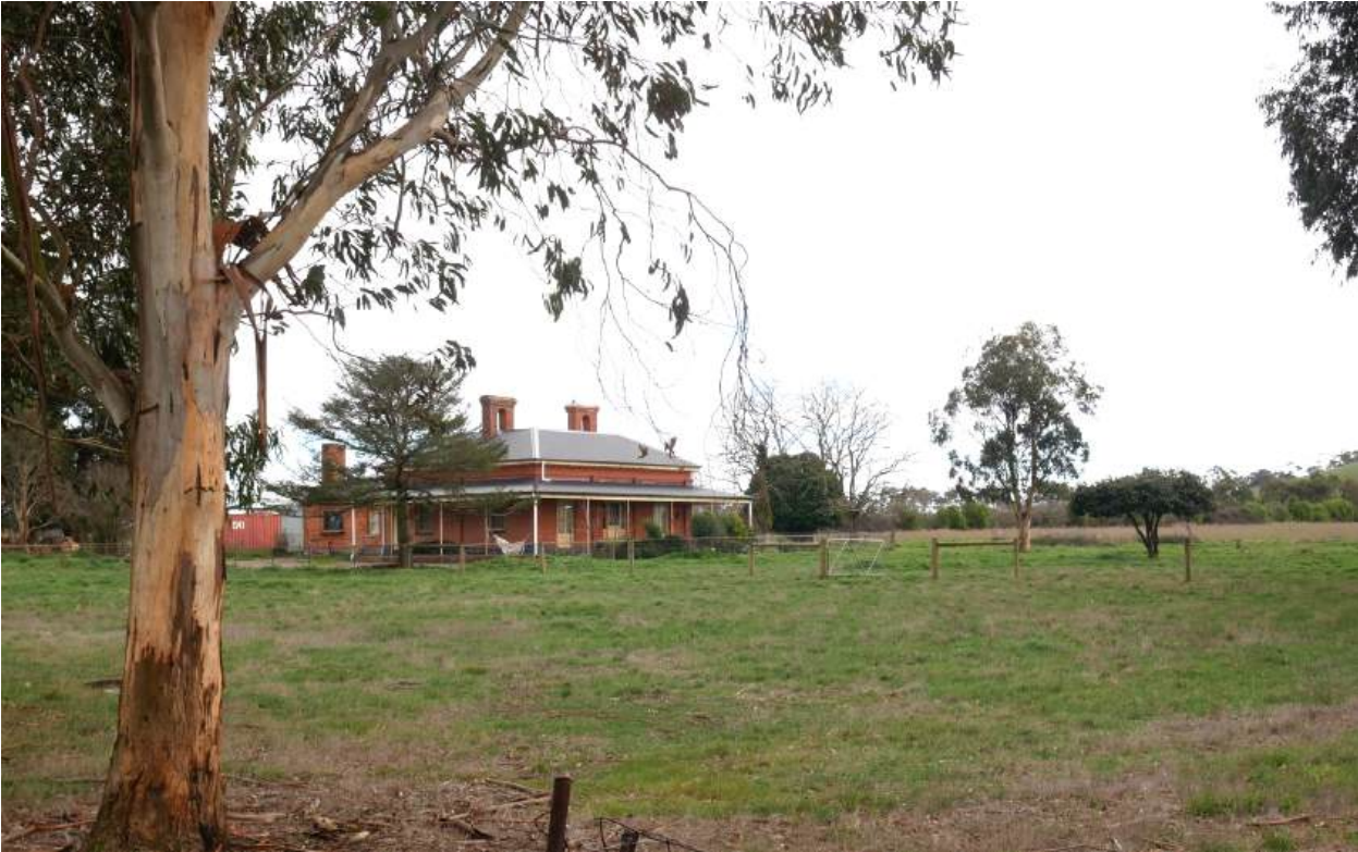
Figure 1. Bernera Homestead from Olliers Road (Source: GJM Heritage, August 2025)
