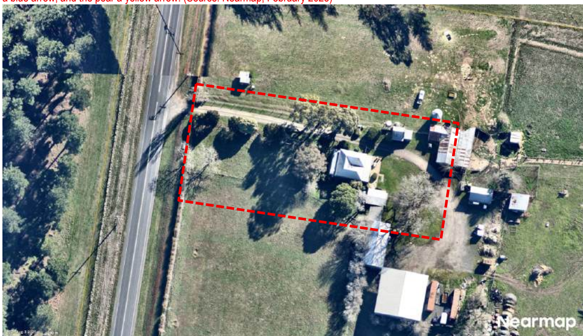
Figure 20. The recommended extent of the heritage overlay for 134 Gillies Road, Mount Rowan, outlined in red. (Source: Nearmap, 3
