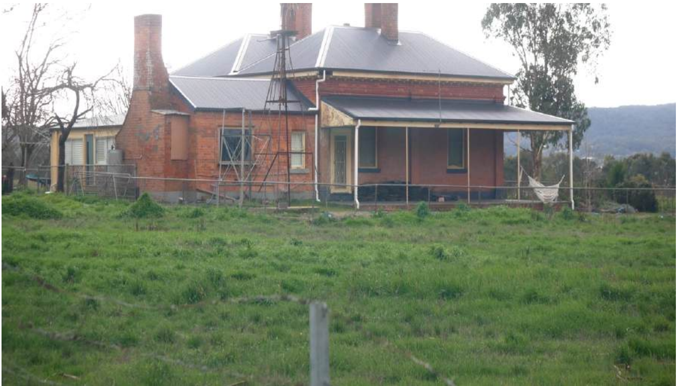
Figure 7. Southern elevation showing rear wing and skillion addition behind (GJM Heritage, August 2025)
