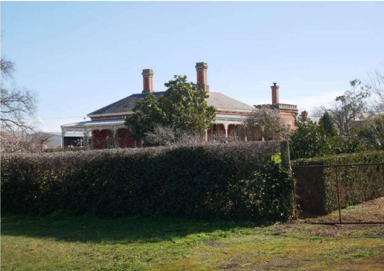
Figure 7. Southern and eastern elevations from Olliers Road (Source: GJM Heritage. August 2025)
