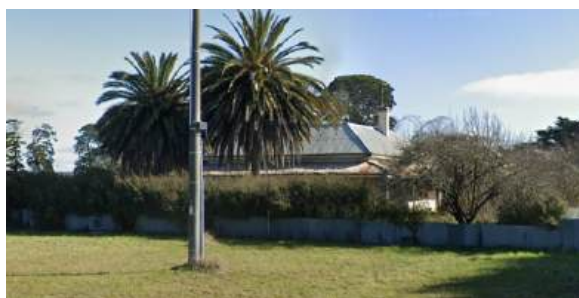
Figure 11. 624 Glenelg Highway, Smythes Creek (Source: Google Street View)
