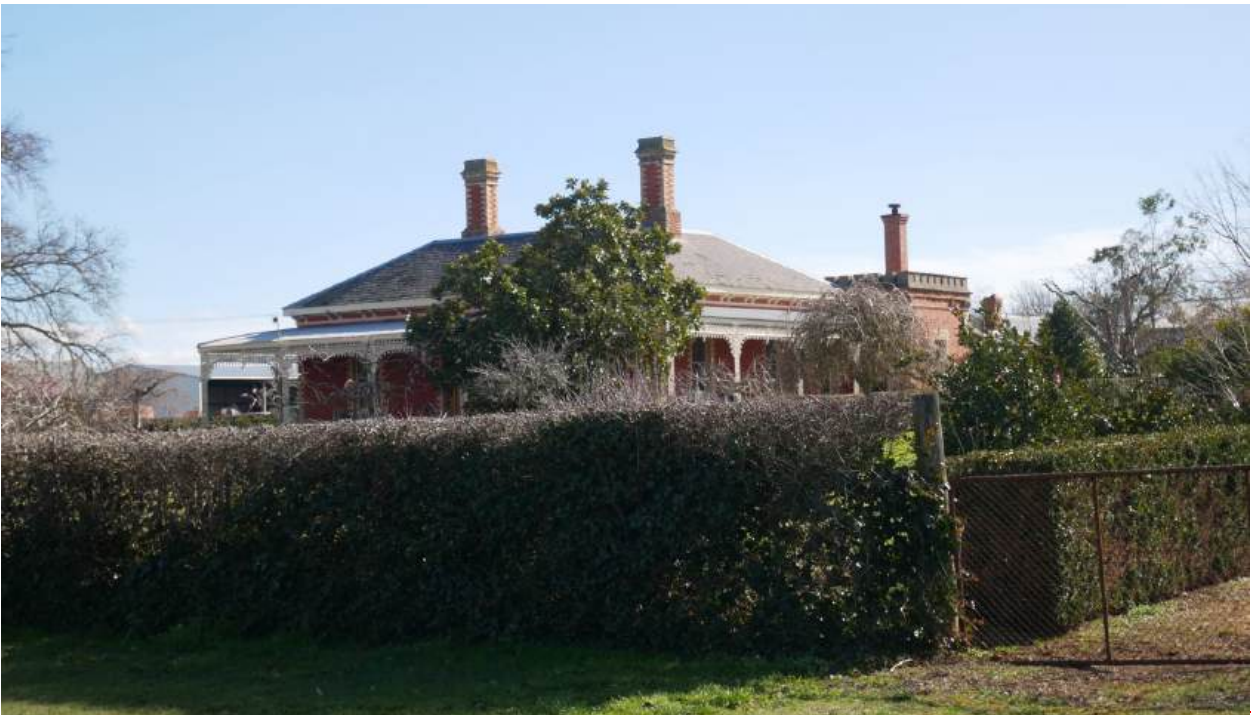
Figure 7. Southern and eastern elevations from Olliers Road (Source: GJM Heritage, August 2025)
