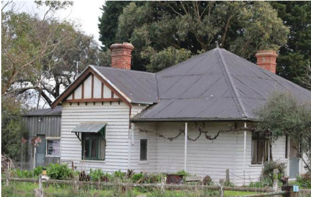
Figures 1 and 2. Scott's Homestead from at 103 Olliers Road – front (north) elevation and east (side) elevation. (Source: GJM Heritage, August 2025; RBA, August 2024)
