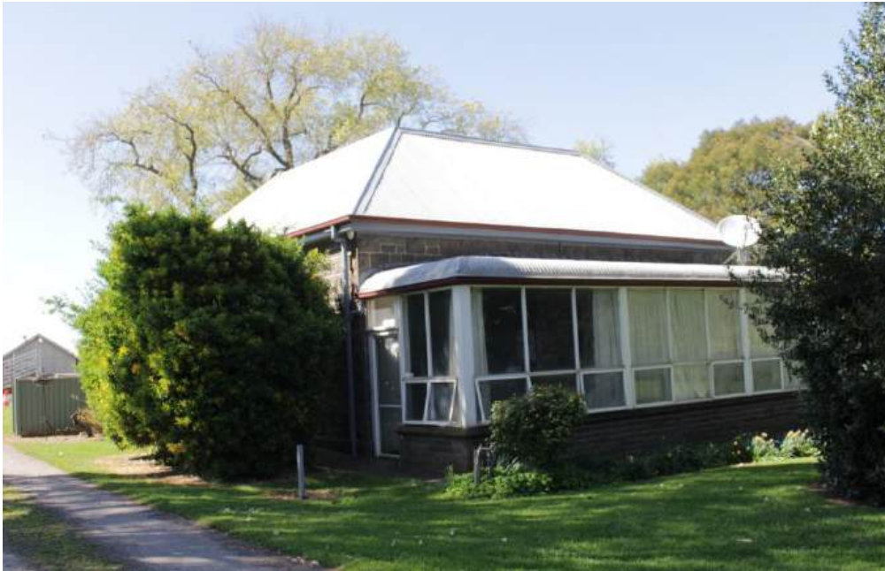
Figure 9. Hawthorn Farm homestead, showing concealed façade (east west elevation) (Source: RBA, September 2023)
