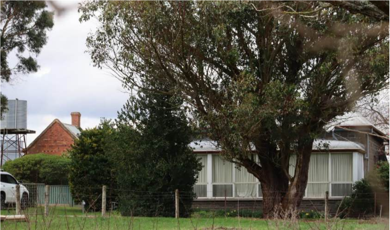
Figure 1. Hawthorn Farm, close-up from Gillies Road, with the brick outbuilding left of frame and bluestone homestead to the right. (Source: RBA, August 2024)
