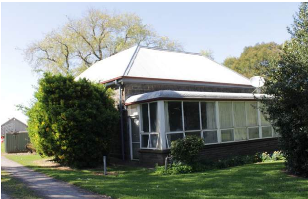
Figure 9. Hawthorn Farm homestead, showing concealed façade (west elevation) (Source: RBA, September 2023)
