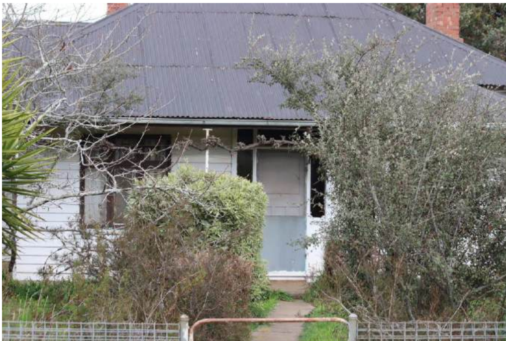
Figure 7. Façade (north elevation) from Olliers Road. (Source: RBA, August 2024)
