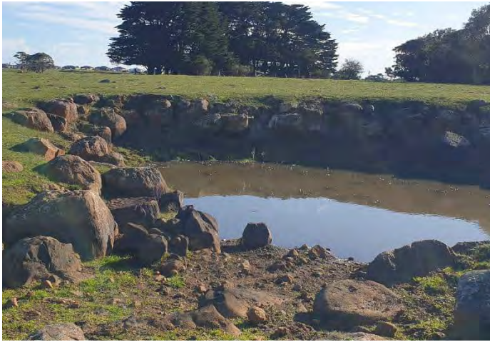
Photograph 6: View of the dam near the eastern boundary of site. The dam is cut into the side of a slope and its walls are primarily basaltic.
