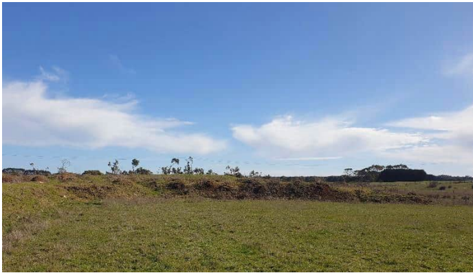
Photograph 50: View facing west of the large area of filling in the south western portion of site. The fill has a varied depth and profile multiple meters deep.
