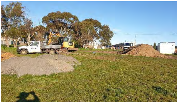
Photograph 78: View facing southeast from the north western portion of site. The western portion of site is used as a depot for a civil contractor, stockpiles of topsoil and crushed rock are visible.
