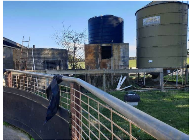
Photograph 43: View of two above ground tanks and a silo adjacent to the stockyards.
