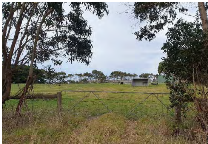
Photograph 92: View facing south from the northern boundary of site. A stockyards and barn can be seen in the right of image. The ground is undulating and has varied grass health, indicating potential filling
