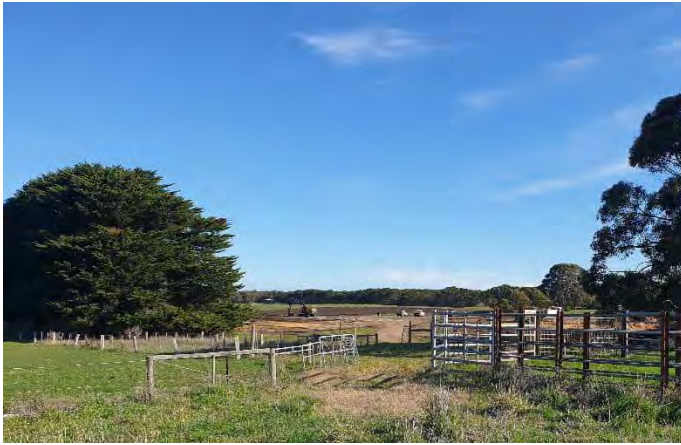
Photograph 17: View of the earthworks in the northern portion of site.
