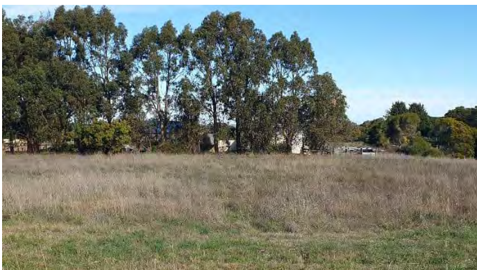
Photograph 15: View facing south of the front of site. A stockyard can be seen in the right of image, and the site office/sheds for the earthworks onsite can be seen behind the tree line.
