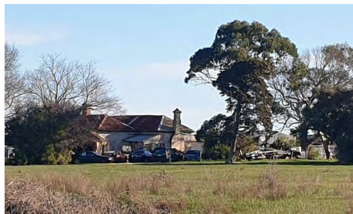
Photograph 34: View facing west of the residences. A stockpile of hard waste, and multiple cars both running and rusted shells are visible.
