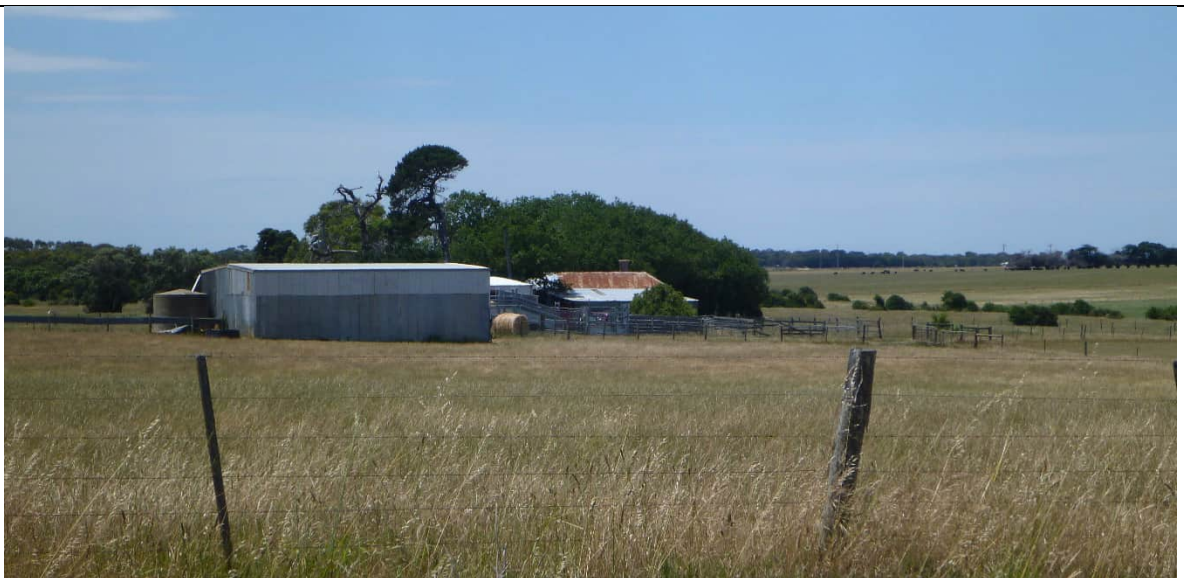
Stockyards and Shedding, 174 Aberline Rd
