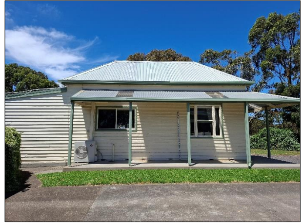
Plate 23: West elevation (side) of dwelling at 75 Rodgers Road (Photograph provided by M. Mirgholami 10.12.2024).
