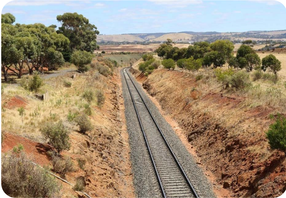
Figure 21. The Ararat rail line which runs through Parwan.
