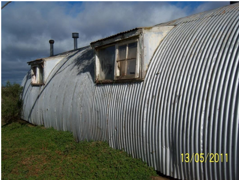
Plate 15: Side view of Nissen Hut along Bridge Road Melton South (Photograph courtesy of S.J. Peters, 13.05.2011)
