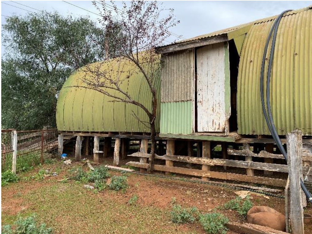
Plate 3: Study area facing south-west showing Nissen Hut at 1232-1290 Beattys Road (Photograph by M. Filihia 12.05.2022)
