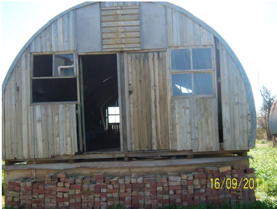
Plate 11: Front and base view of Nissen Hut in a farm on Ferris Road utilised for grain storage (Photograph courtesy of S.J. Peters, 16.09.2011).
