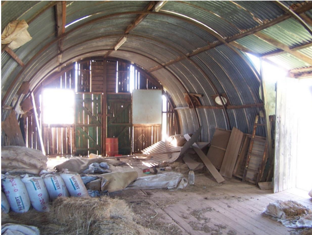
Plate 13: Front and base view of Nissen Hut in a farm on Ferris Road used for storage (Photograph courtesy of S.J. Peters, 16.09.2011).
