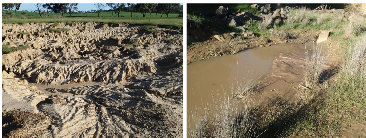
Figure 2-2. Example of erosion of sodic and dispersive soils which can result in elevated turbidity and sedimentation in waterways.
