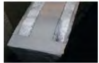
Asbestos thermal insulation (friable)
