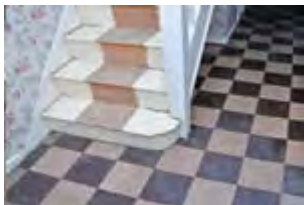
PVC or vinyl floor tiles with added asbestos (low %) chrysotile (non-friable)
