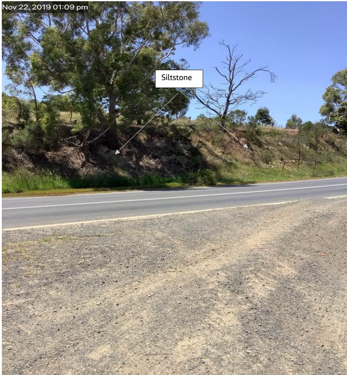
Figure 5-2. Siltstone and residual soil along the Darraweit road
