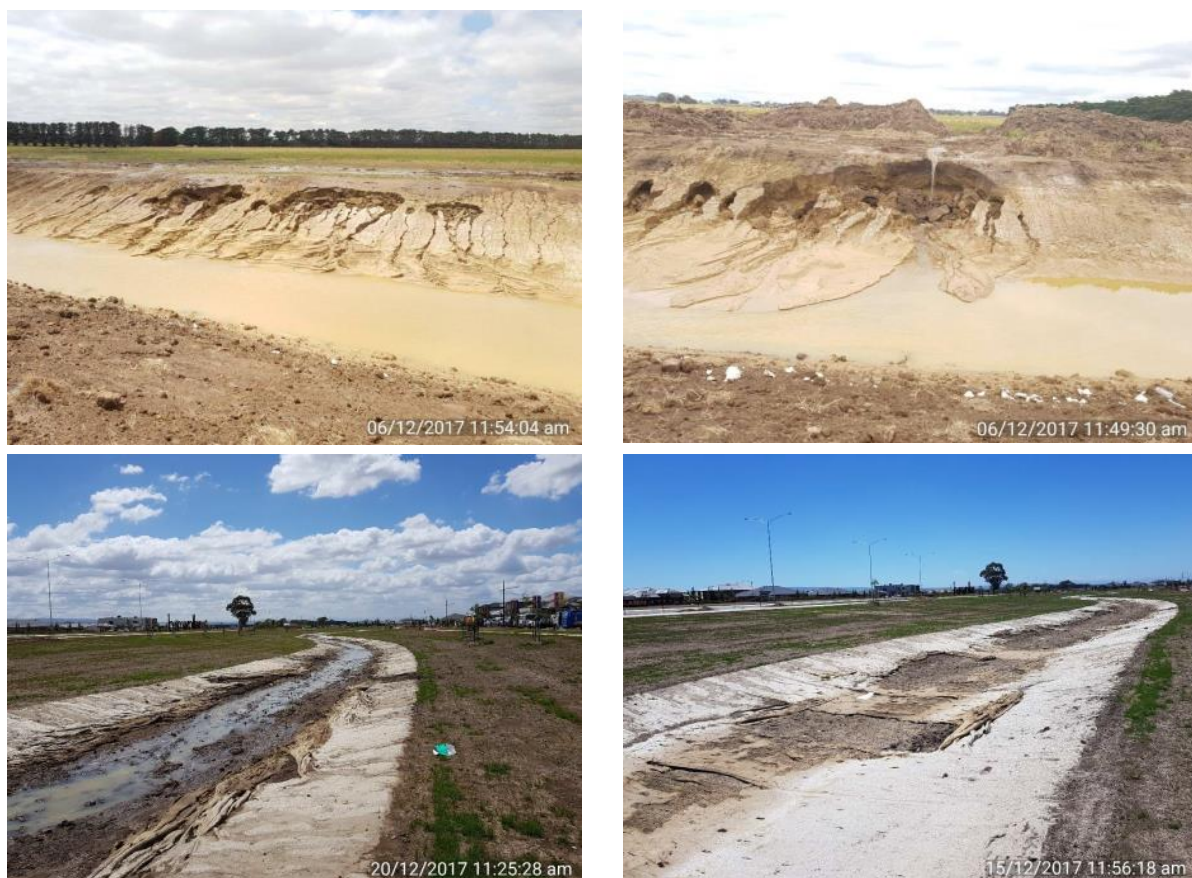
Figure 5-7. Selected photographs of erosion and damage to drains at Merrifield following rainfall events (Brizga & Seymour 2018).
