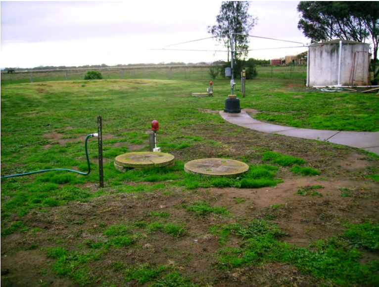
Photo A.1 : Waste water drain covers (foreground), Septic tank (background). Property 4.
