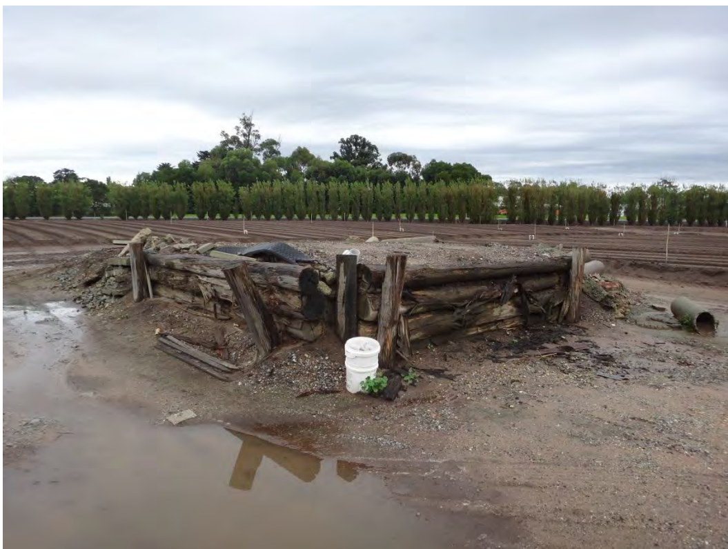
Photograph 136: Dirt hardstand/loading platform located to the south of the processing sheds.
