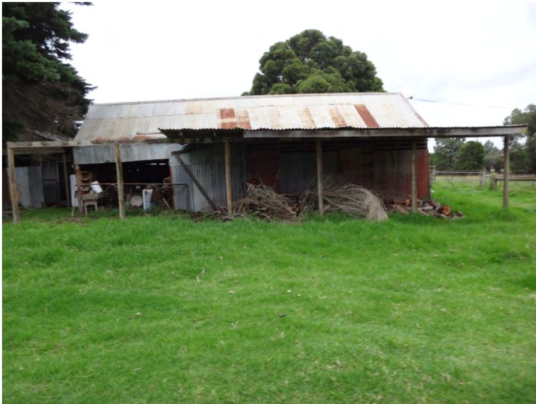
Photograph 10: View west of old farm/storage shed.
