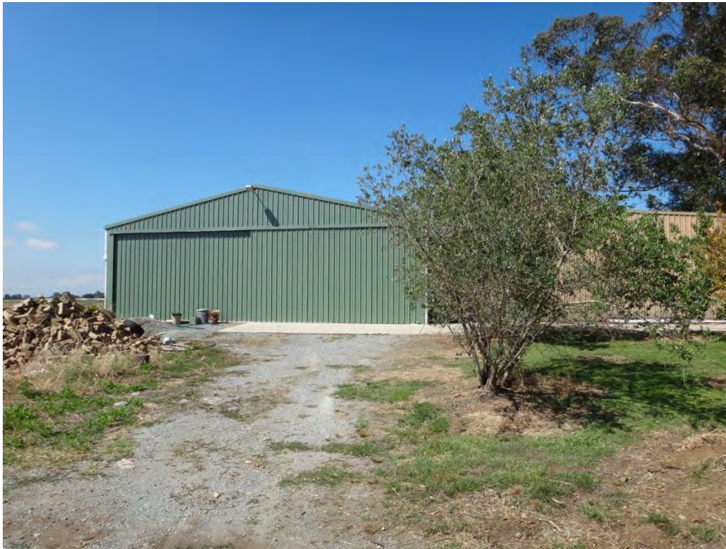
Photograph 59: Storage sheds and woodpile south of the car storage area.
