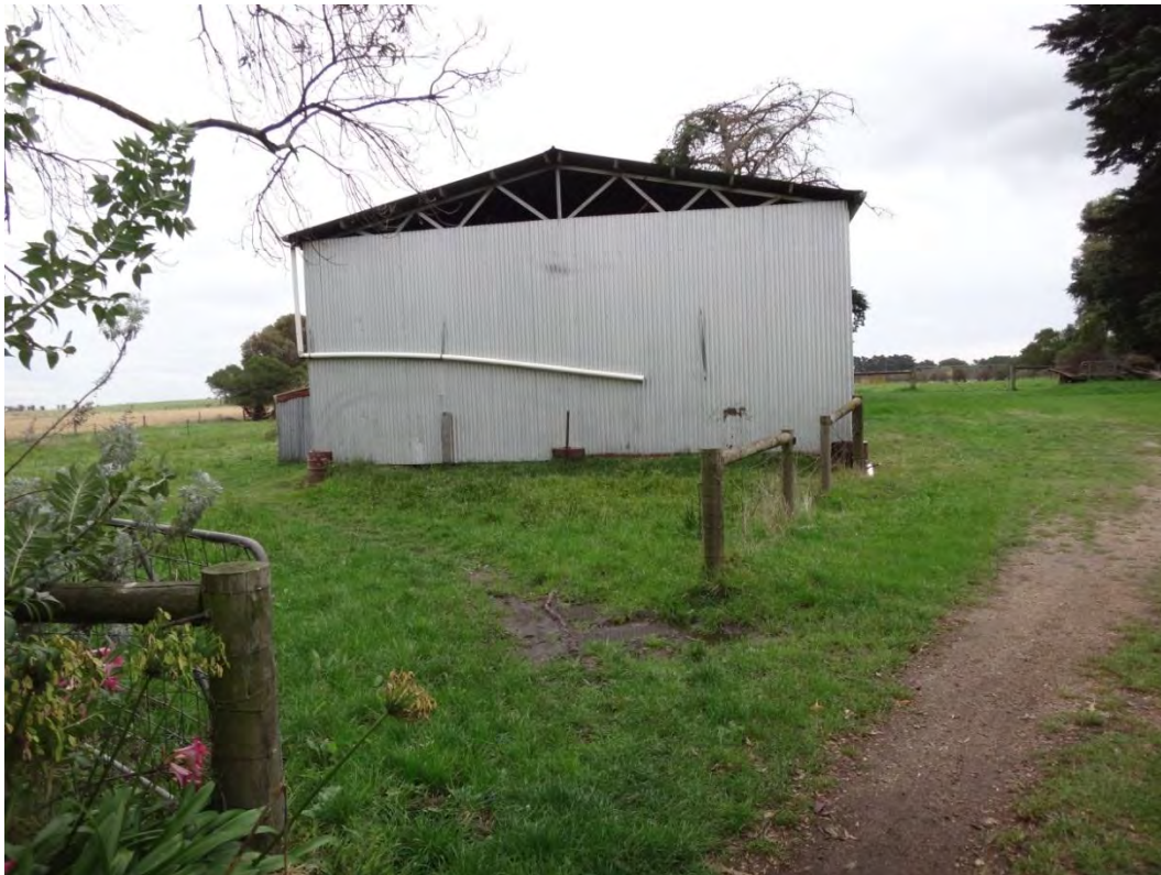
Photograph 11: View south of hay shed.
