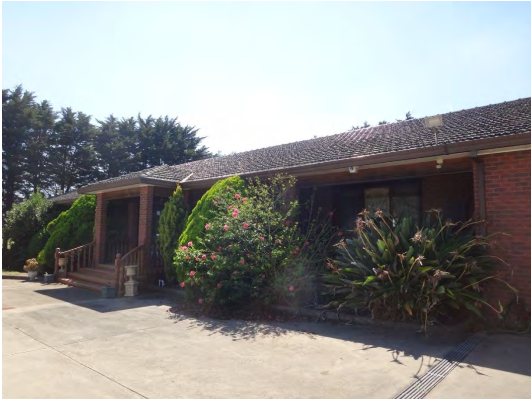
Photograph 55: Concrete driveway and brick residence.
