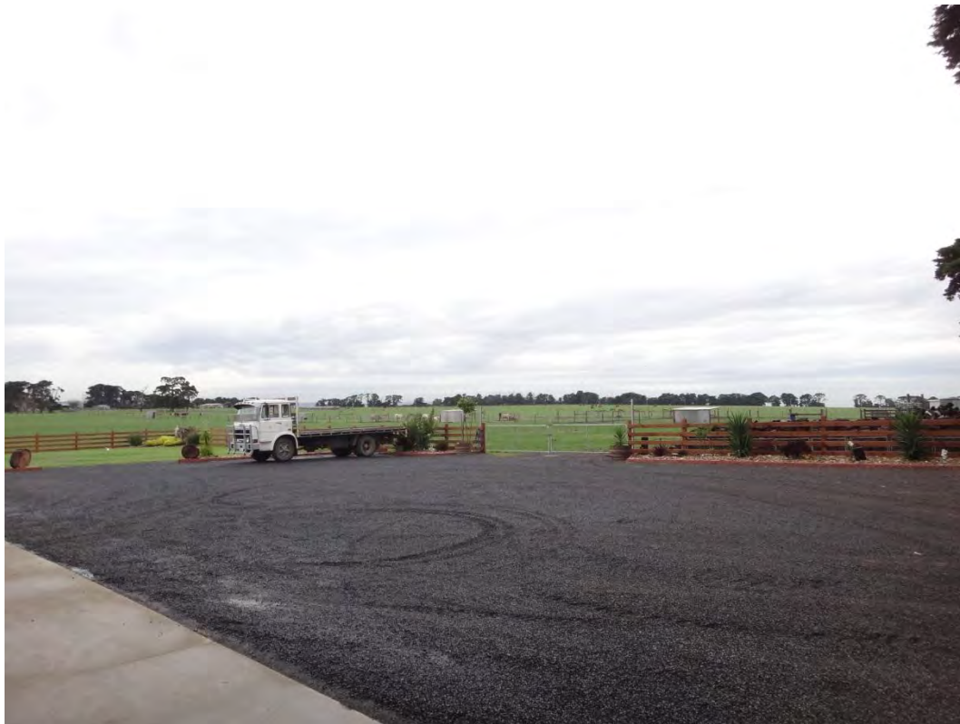
Photograph 17: View east from outside front storage/garage of crushed rock hard stand area.
