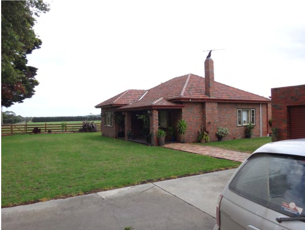
Photograph 15: View north west from Hardy's Road of residence.
