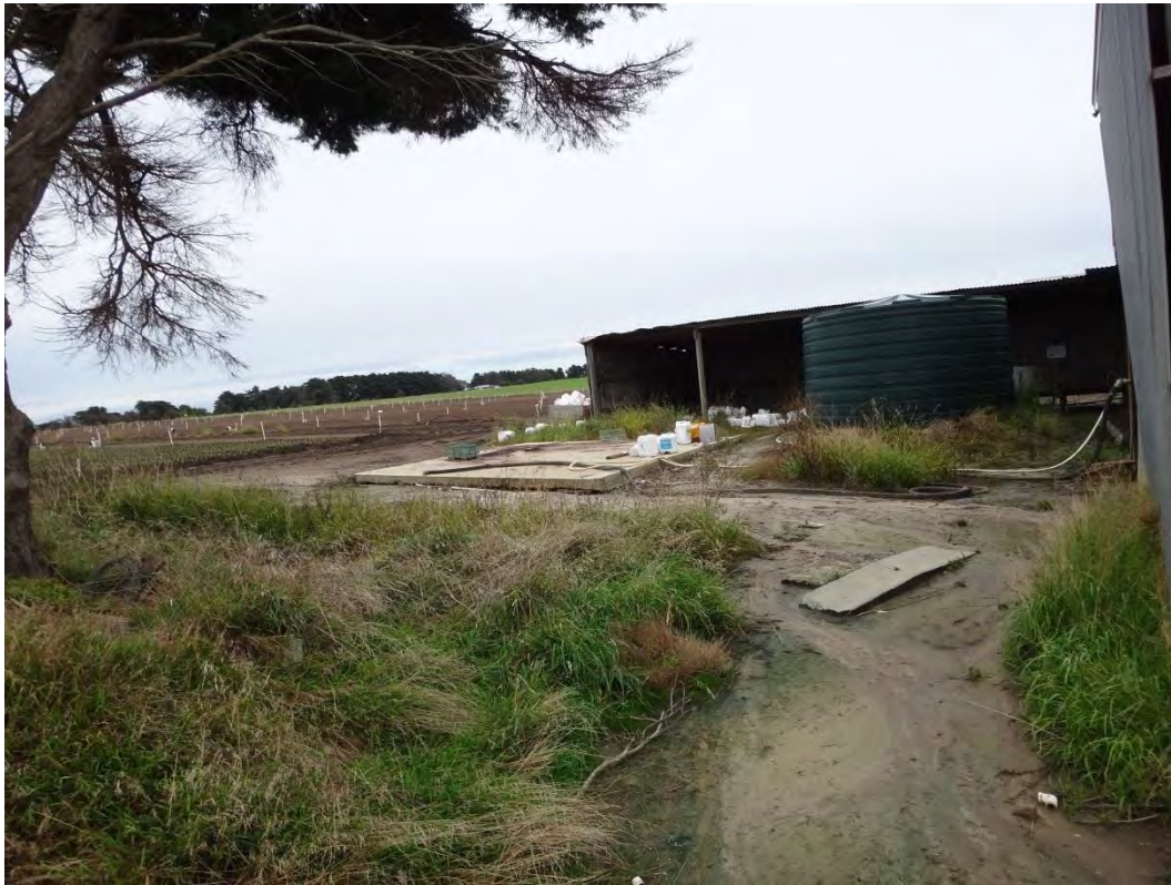
Photograph 139: Concrete hardstand, water tank and chemical storage area in the north portion of the site behind the storage/processing shed.
