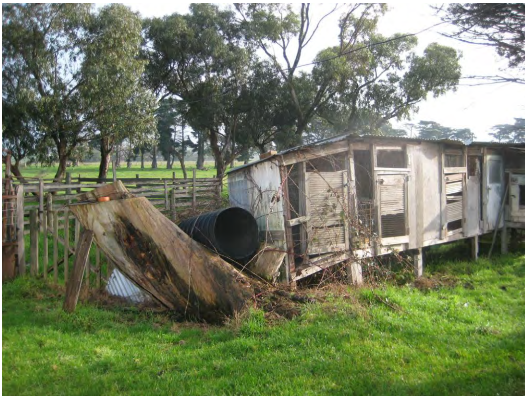
Photograph 146: Old poultry coup located to the west of the brick storage shed.
