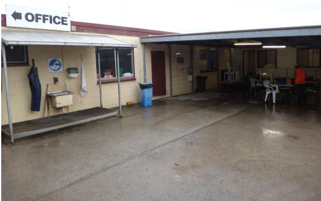
Photograph 132: Office area and staff lunch rooms in the south portion of the property.
