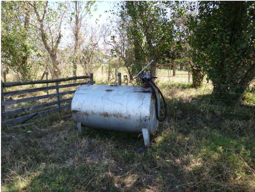
Photograph 66: Diesel AST located to the south of the storage shed.
