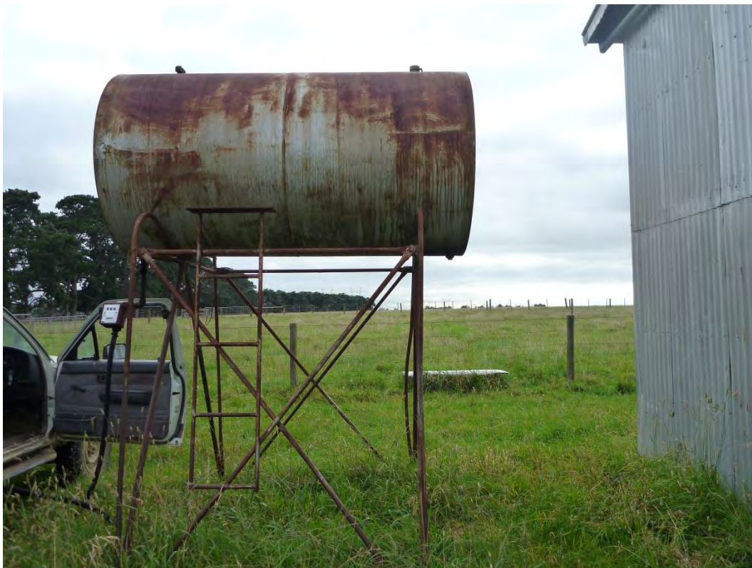
Photograph 25: AST located north of former milking shed.
