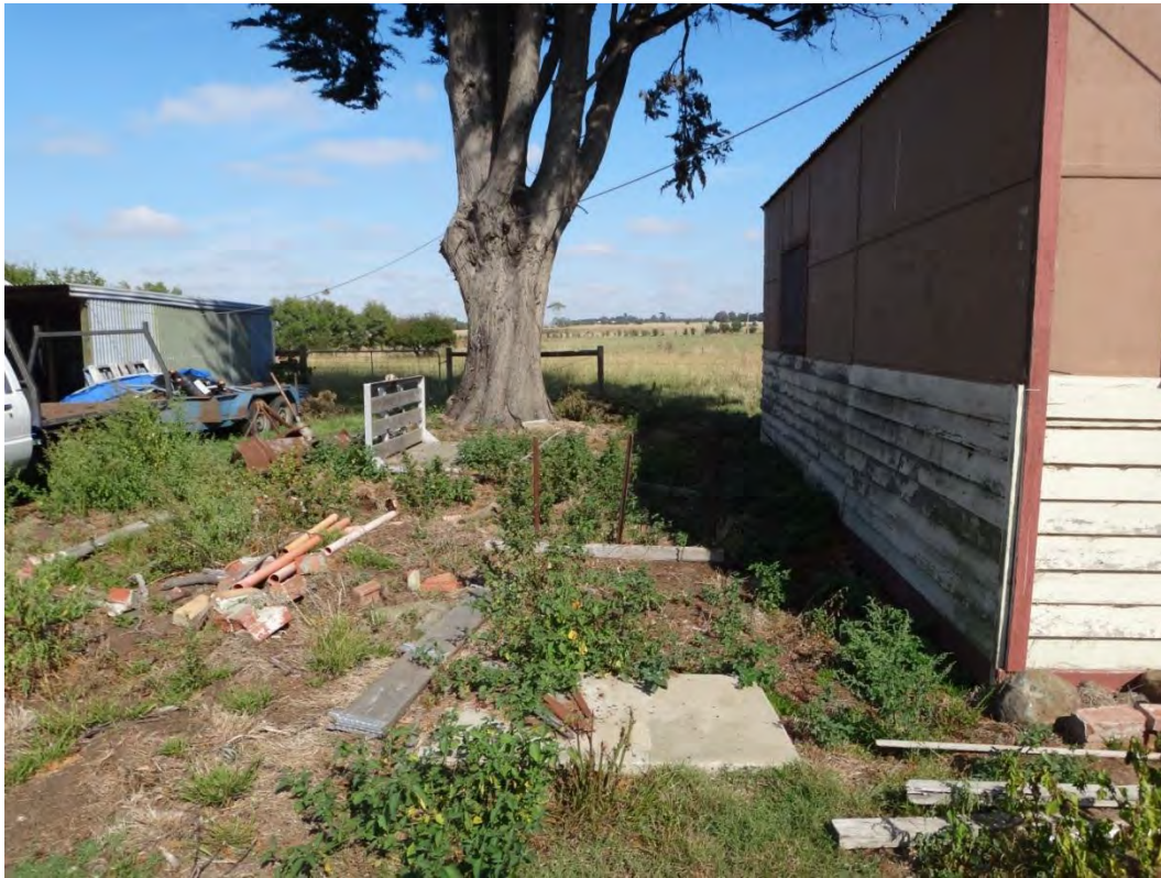
Photograph 54: Area of disturbance/demolished building west of residence.
