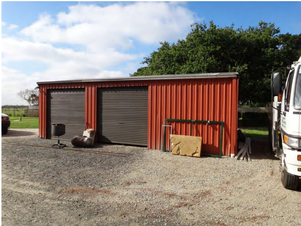
Photograph 46: Storage shed/entertainment room north of residence.
