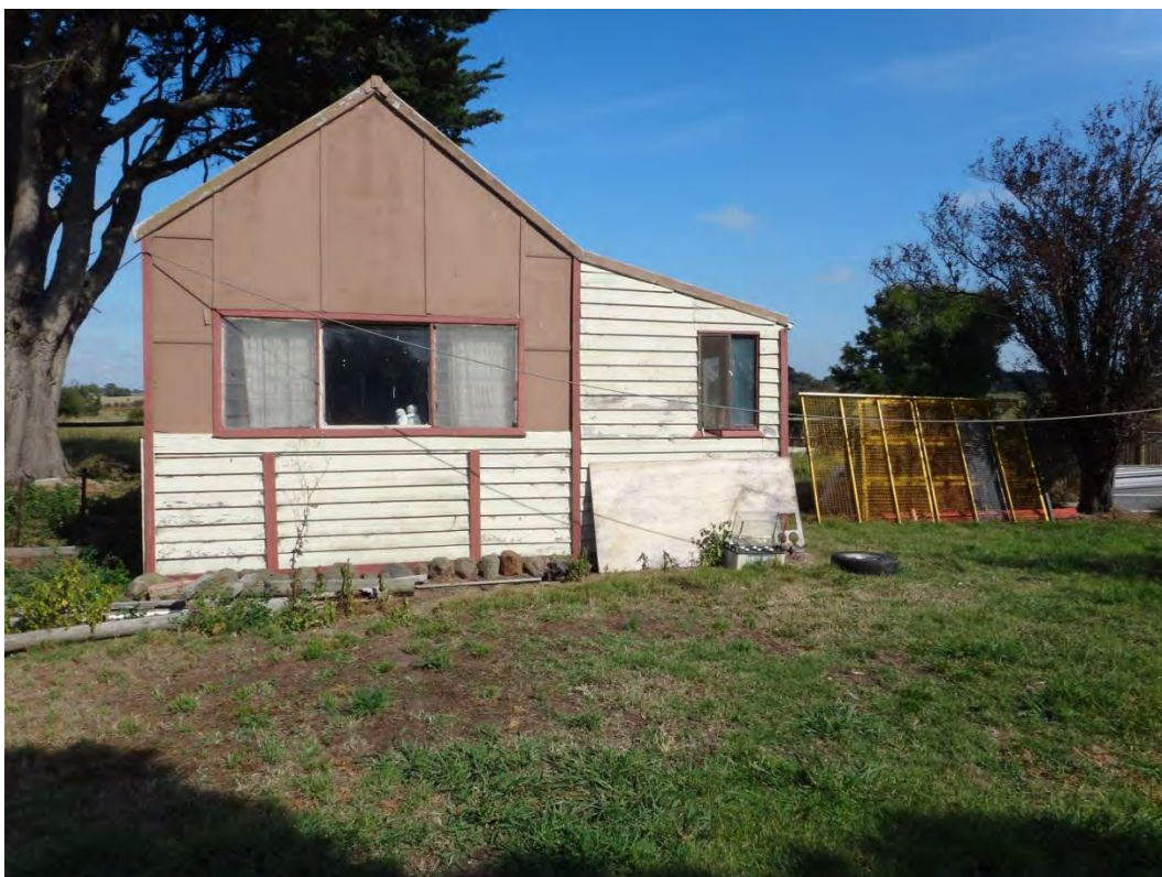
Photograph 53: Weatherboard and bonded cement storage/entertainment shed west of residence.
