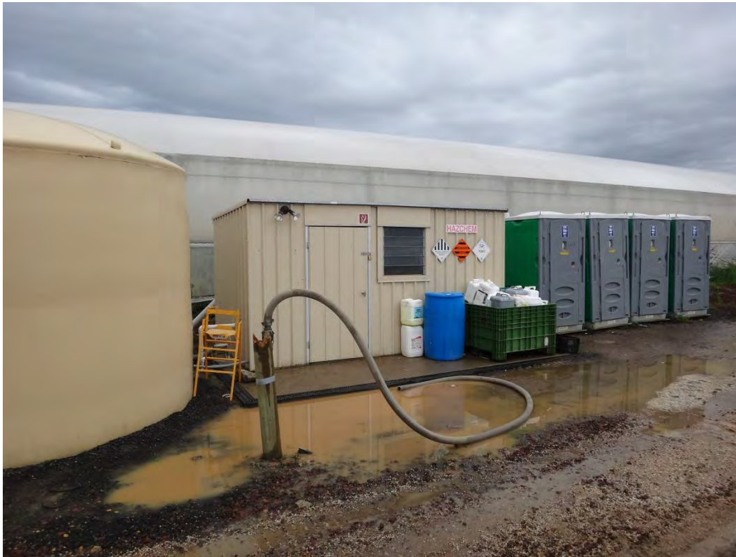
Photograph 151: Water tank, groundwater bore and chemical storage shed located adjacent to greenhouses in the south portion of the property.
