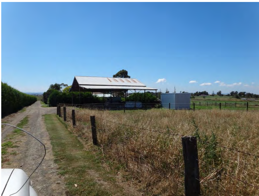
Photograph 78: Hay and vehicle storage shed located north of the former milking shed.
