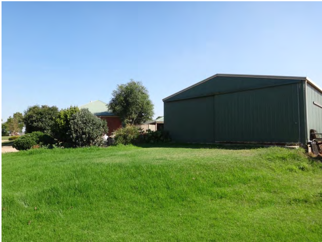
Photograph 94: Storage shed along east property boundary.
