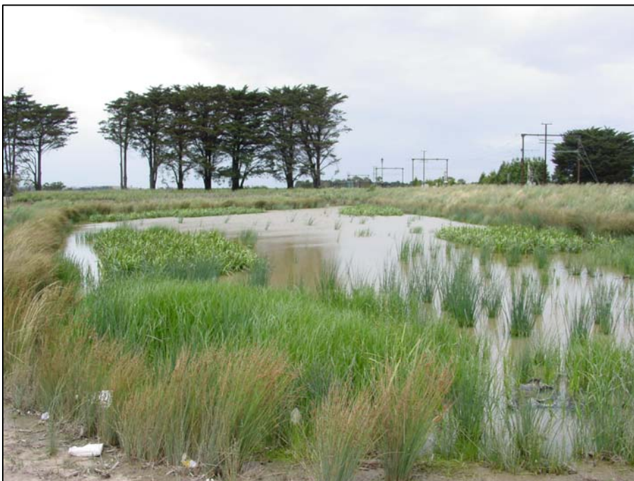
Plate 4. Recently constructed wetlands planted out with a diversity of wetland plants, Pakenham, Victoria.
