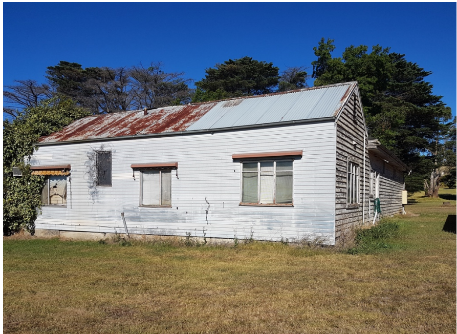
Figure 5 The workers' quarters as viewed from the west. This elevation has been reclad and its fenestration appears to have been altered.
