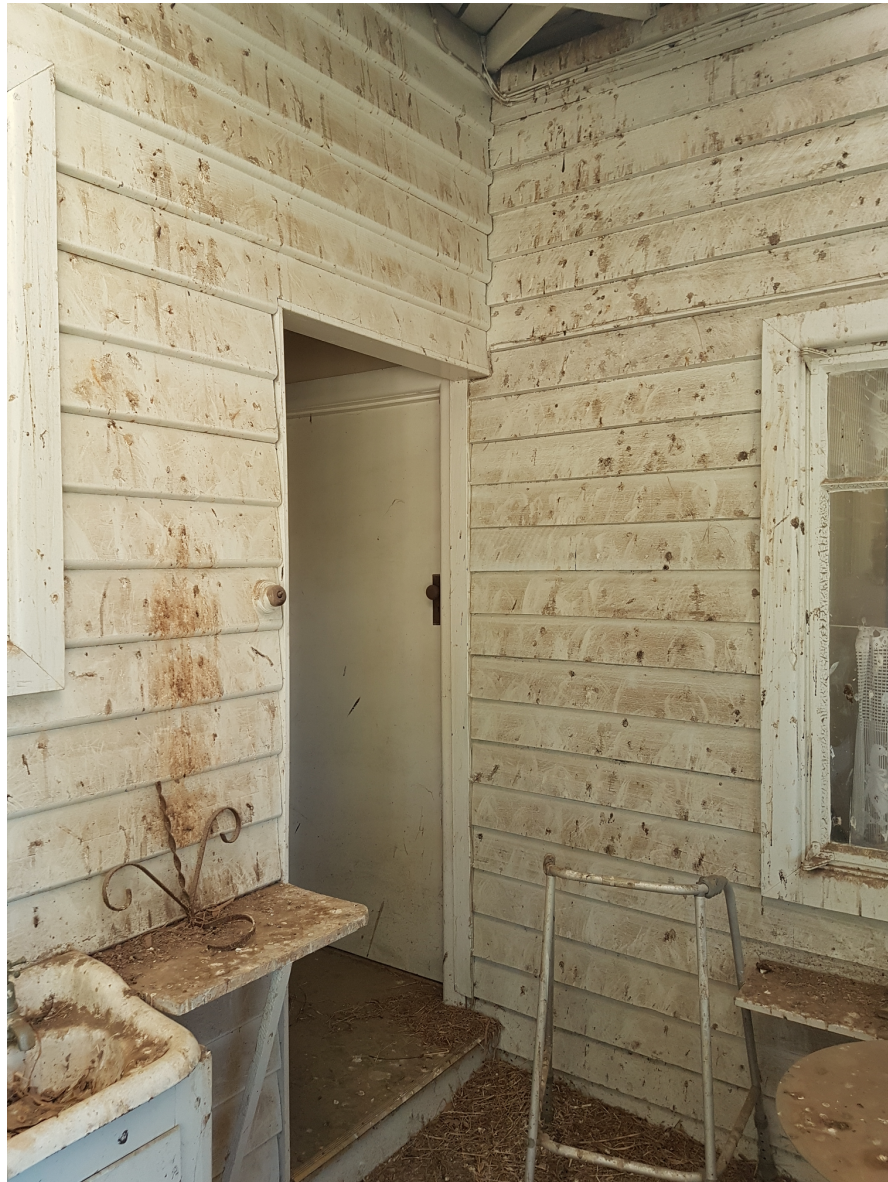
Figure 8 The two wings of the workers' quarters appear to be butted together with an awkward junction to both walls and breezeway roof rather than constructed in a conventional sense. The two different board profiles are also evident in this view.
