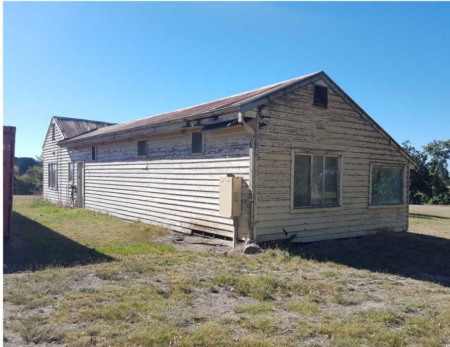
Figure 6 View of the workers' quarters from the south. Note the highlight louvred windows to the left, and the altered or atypical single pane window to the right.
