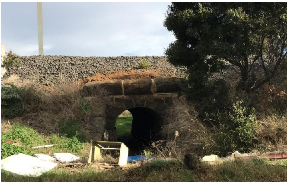
Figure 3 – Existing Railway Culvert
