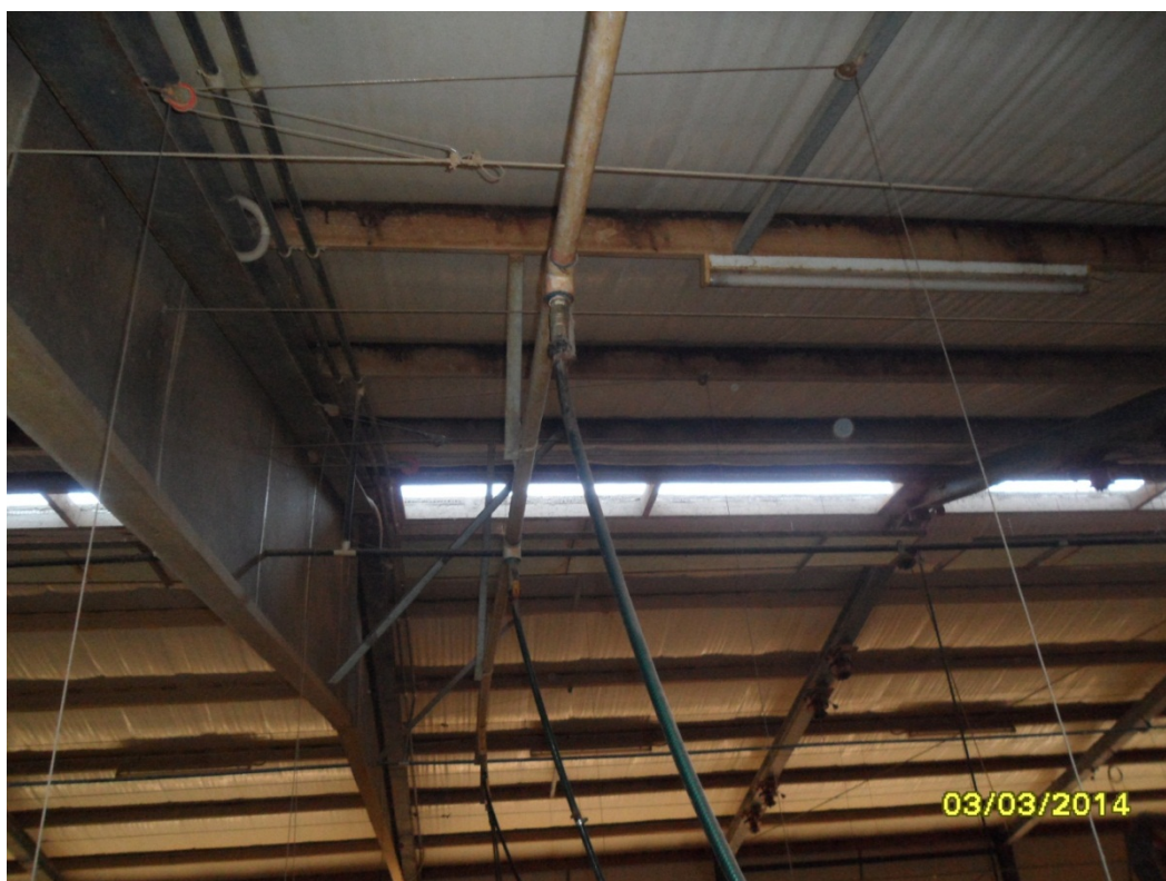
Figure 5 Shed ceiling showing fogger lines and ridgeline vent
