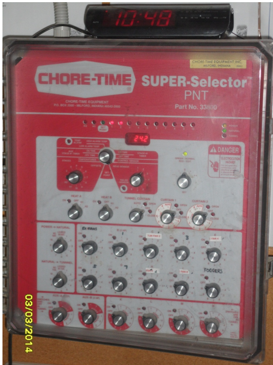
Figure 7 Vent Aperture, fogger and gas heater controller.
