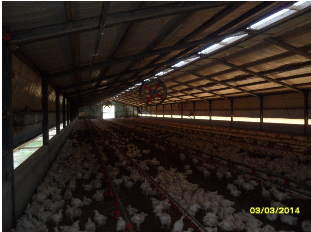
Figure 6 Inside of Shed showing stirring fans, concrete side wall, side slots and ridgeline vent. Note lowered feeder and nipple drinker lines and opened end door
