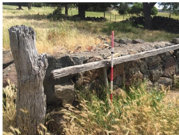
Plate 42: Looking south west, stock ramp constructed of basalt, bluestone, brick and concrete
