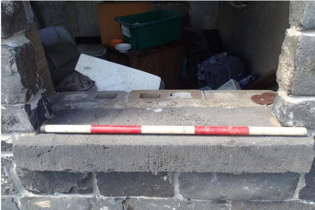
Plate 69: Window in repaired section of north wall. Note breeze block reinforcement
