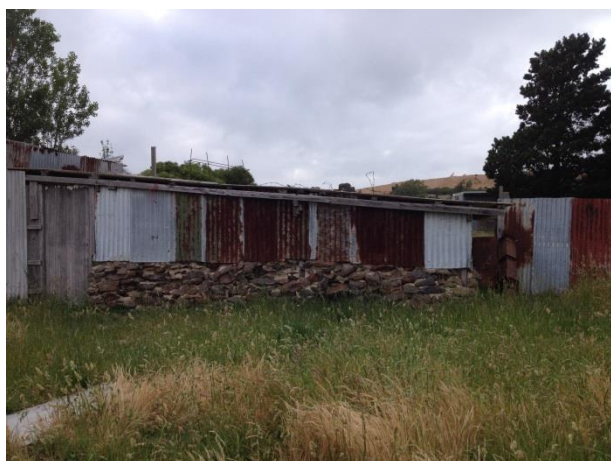
Plate 7: Looking east, basalt rock and corrugated iron shed used for pig husbandry, 90 Langley Park Drive.
