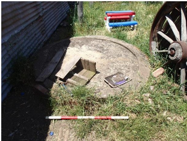
Plate 61: Looking south, red and cream brick-lined well sealed with concrete
