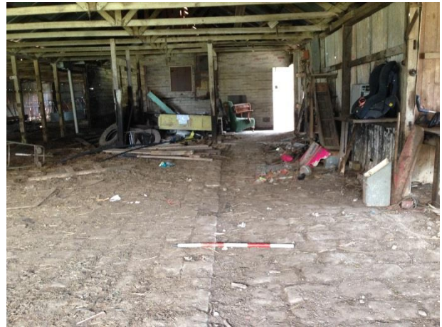
Plate 26: Looking north, bluestone flagged floors in milking shed
