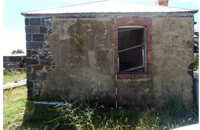
Plate 70: Looking east, west-facing wall of cottage with brick rowlock arch window and lime plaster
