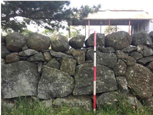
Plate 45: DSW16, southern elevation, looking north, showing well graded stone courses and fine stone placement
