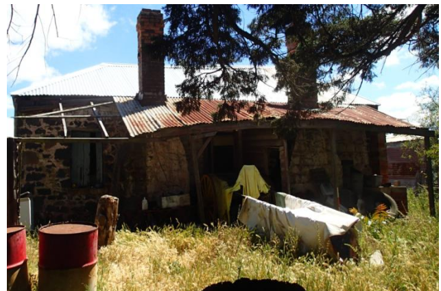
Plate 72: Looking north, view of bluestone and brick chimneys in south wall of cottage
