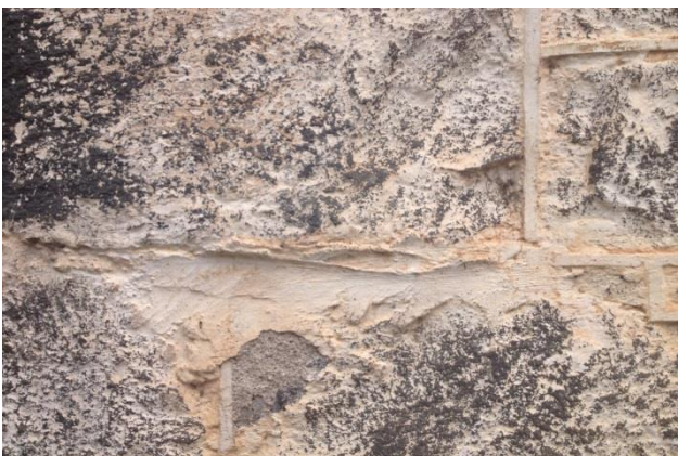
Plate 73: Detail of east wall showing lime wash over bluestone
