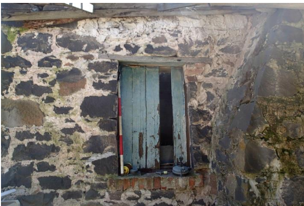
Plate 71: Looking north, timber window in south wall of cottage with red brick lintel
