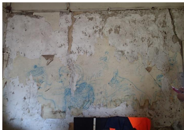
Plate 78: Drawings on western internal wall in Room 2 showing wall paper and lime plaster
