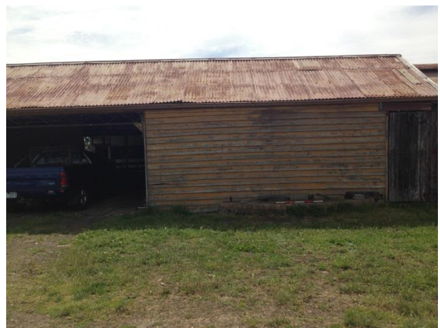
Plate 28: Looking west, timber and corrugated iron garage. Note brick feature at base of wall
