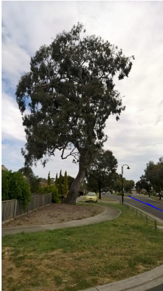
The above is of a River Red Gum in Lake Boulevard, South Morang, a road built some 12 years ago. According to the Council TPZ specs., there should have been no excavation closer to the tree than the blue line. In reality, the excavation has taken place even within the Aust. Std. guidelines.
