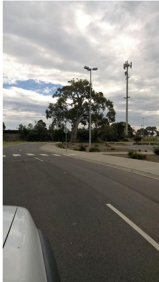
The above road was built through paddock at Lyndarum estate some 5 years ago. According to the Council TPZ specs., there should have been no excavation closer to the tree than well past the kerb.
