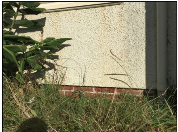
Figure 10: Eastern Façade – roughcast finish detail
