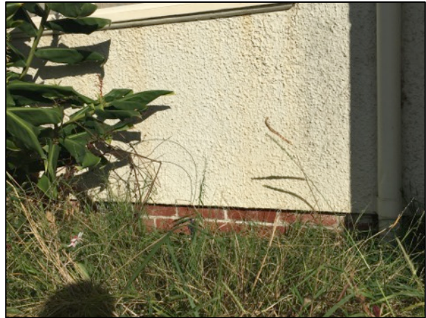
Figure 7: Eastern Façade – roughcast finish detail
