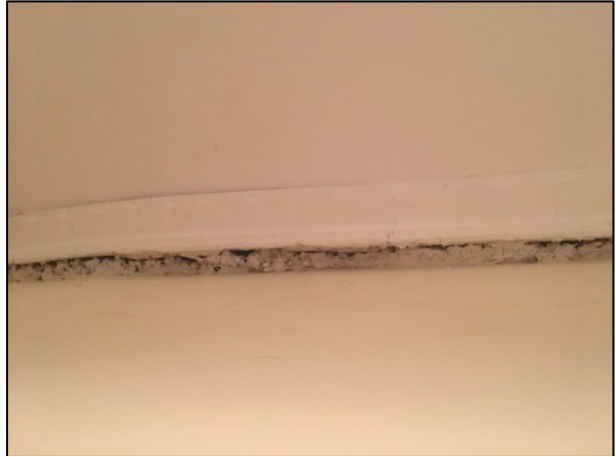
Photo N: Internal - water damage – western bedroom
