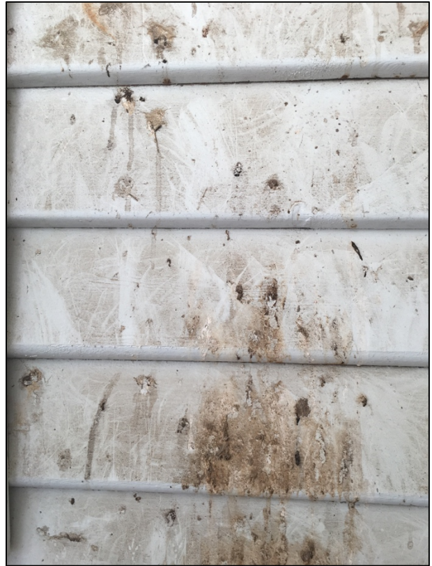
Figure 18: Bull – nosed weatherboards (front wing)
