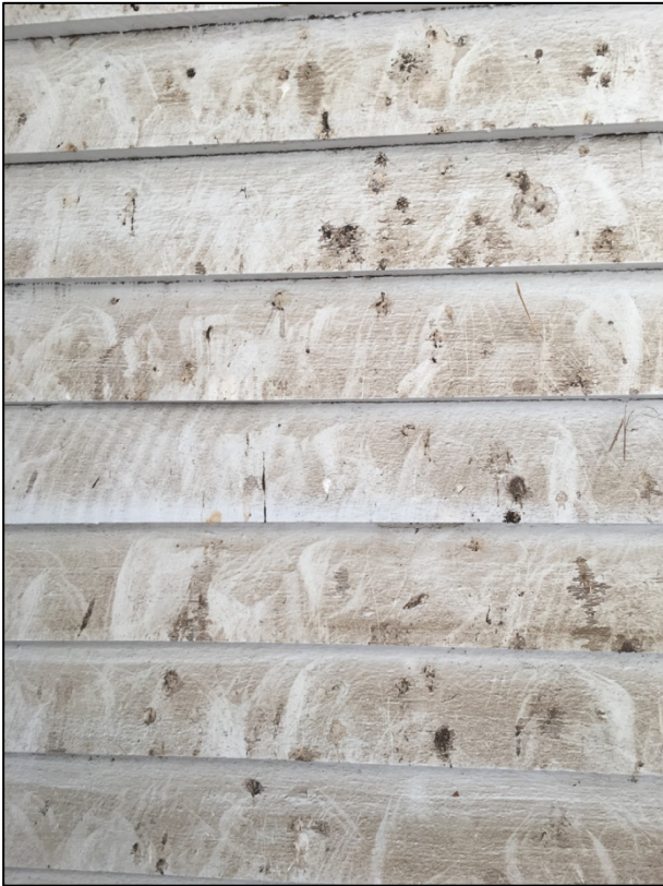
Figure 17: Square – edged weatherboards (rear wing)
