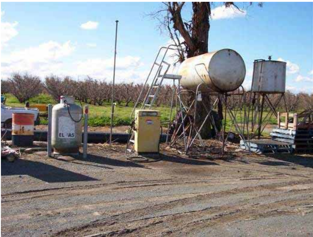
Plate P8: 139 Grahamvale Road - AST containing diesel and dispenser
