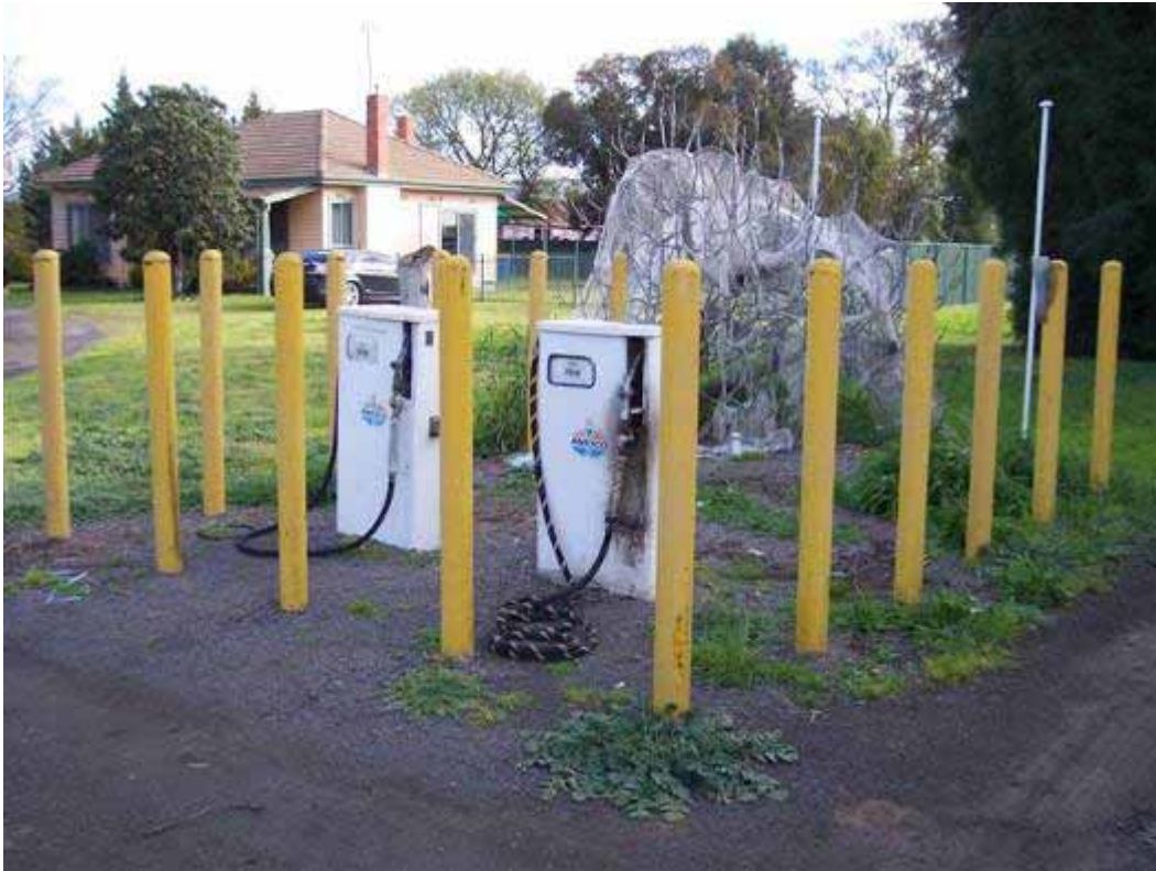
Plate P7: 65 Grahamvale Road - Barricaded dispensers and possible UST
