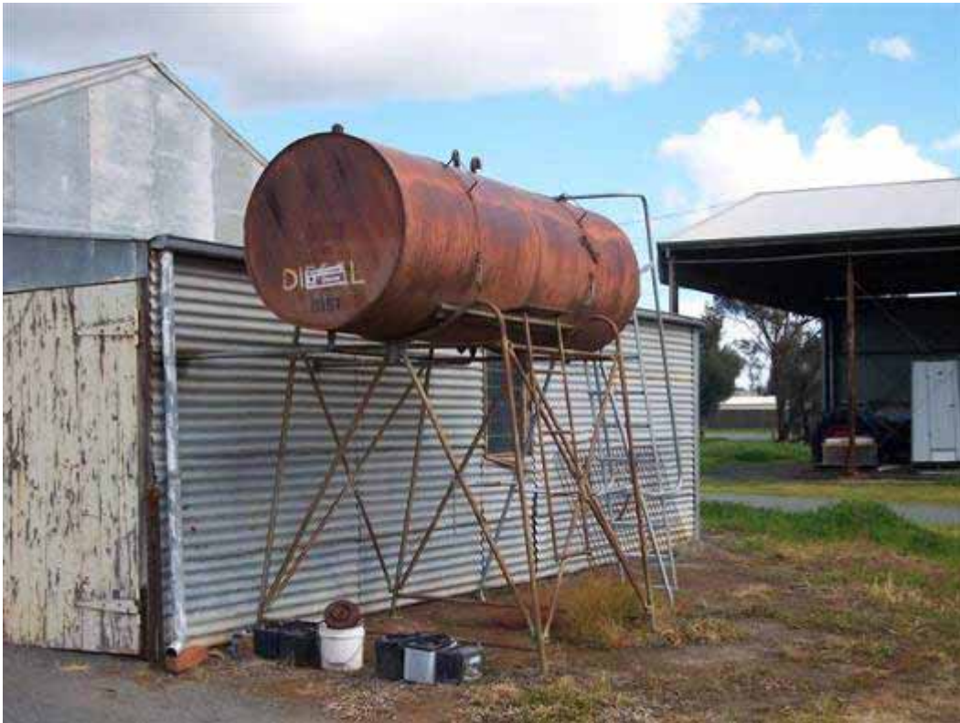
Plate P15: 185 Verney Road - AST containing diesel with automobile batteries stored on ground
