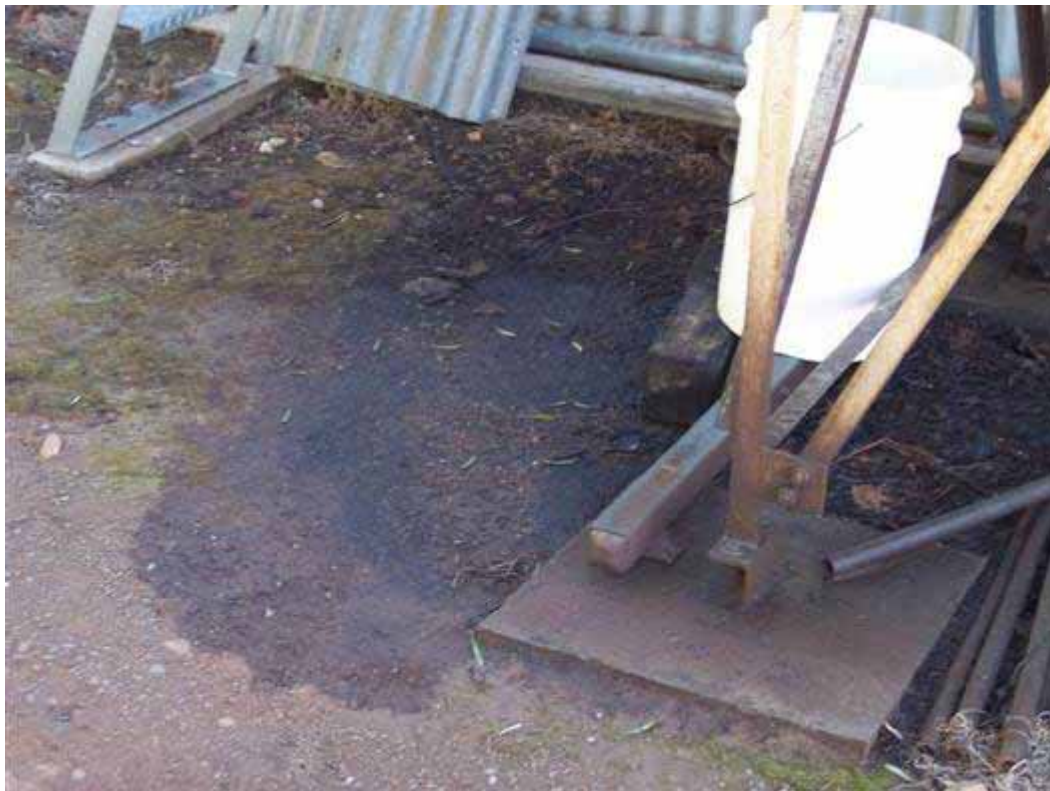
Plate P22: 240 Ford Road - Close-up of ground staining beneath AST
