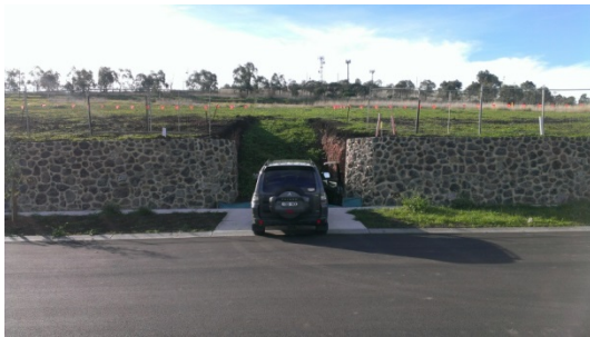
High Retaining walls with step driveways
