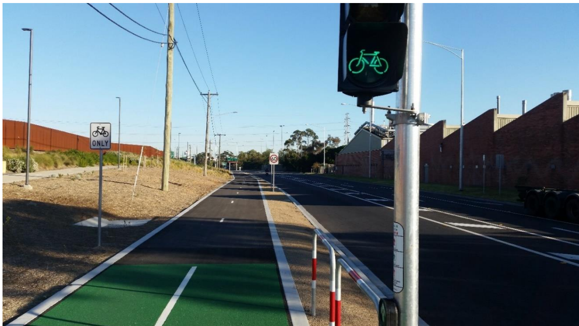
Figure 10: Todd Road, Port Melbourne Example of Secondary Arterial Road with two-way off-road bike path
